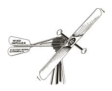
To showcase their capabilities, the Wind-Impeller Electric Works of Ellsworth erected a demonstration outfit atop a 75-foot steel tower. This impressive structure featured a 2400-watt generator, which was primarily sold more in areas east of Ellsworth.
